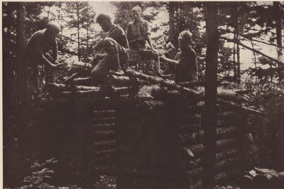
CABIN UNDER CONSTRUCTION
