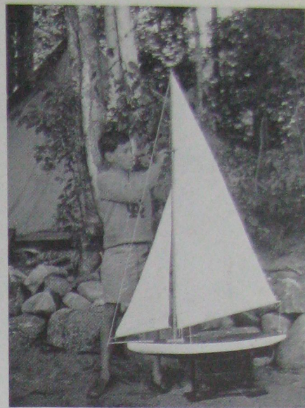
Taller Than He Is A 30-Inch Model Which Sails Nearly as Fast as Its "Skipper" Can Row. It Has a Heavy Lead Keel, Hollow Hull and Pine Spars
