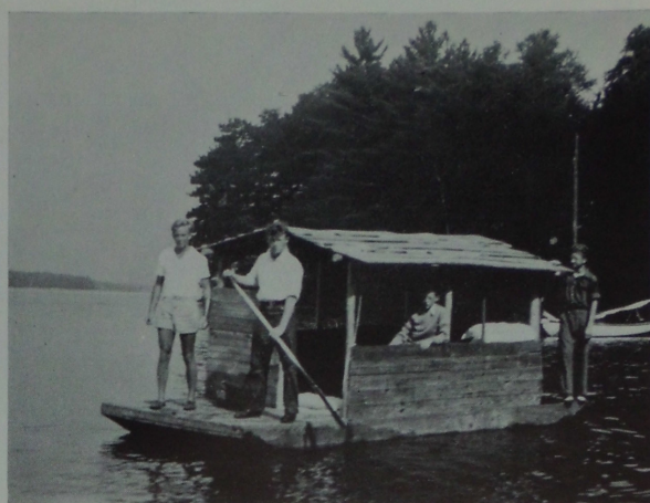
HOUSEBOAT BUILT BY MASTER CAMPERS It was thoroughly calked, made water-tight, and equipped with four bunks. The boys anchored it to a reef and slept in it several nights during the season.
