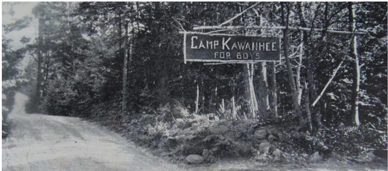
The original camp sign, the camp road is to the right and the dirt road is Route 142 before it was paved.
