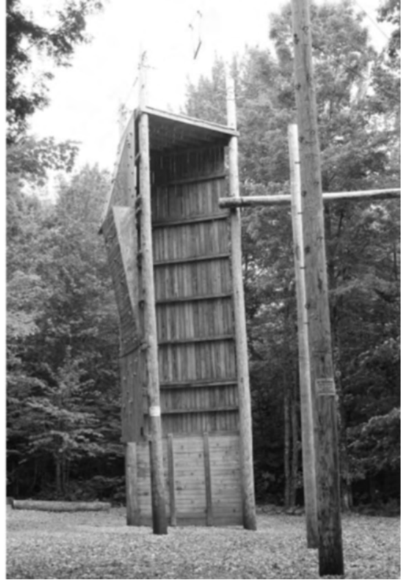
The new Ropes Course and Climbing Wall was made possible by a generous donation from the Abbott family.
